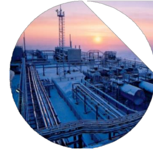
Monitoring of various infrastructures
